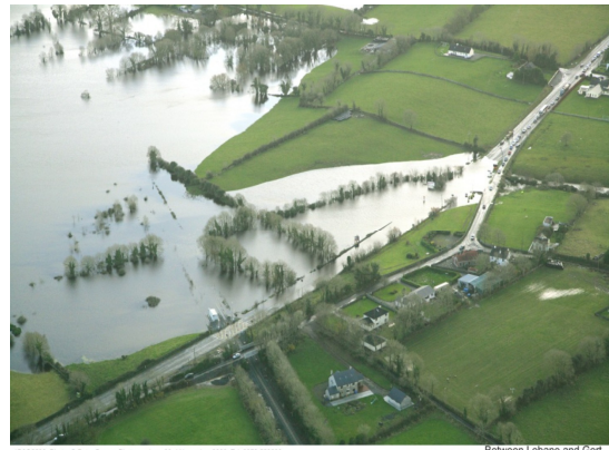
10205530 Photo: © Peter Barrow Photographers 23rd November 2009. Tel: 0872 559638 Between Labane and Gort Flooding N18 at Labane
