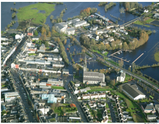
10205414 Photo: © Peter Barrow Photographers 23rd November 2009. Tel: 0872 559638 Ballinasloe Flooding Ballinasloe Town
