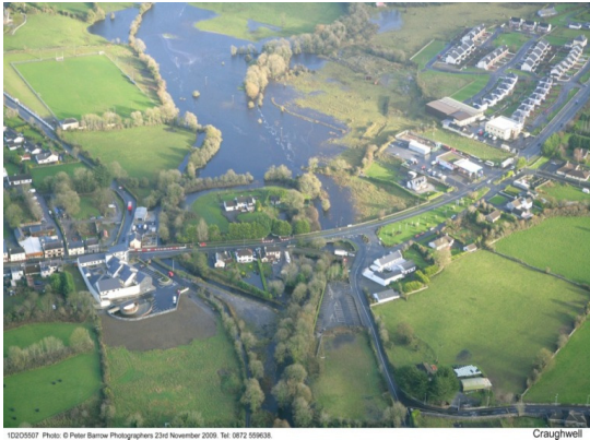
10205957 Photo: © Peter Barrow Photographers 23rd November 2009. Tel: 0872 559638 Craughwell Flooding N6 at Craughwell
